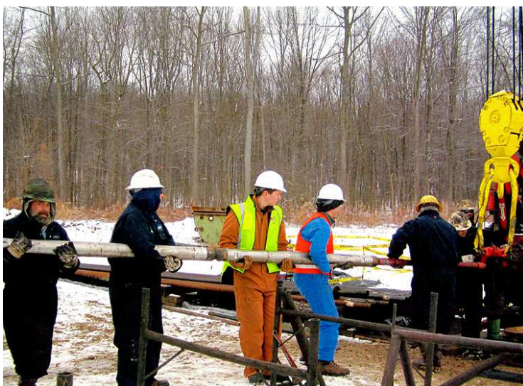
Borehole seismometer installation
